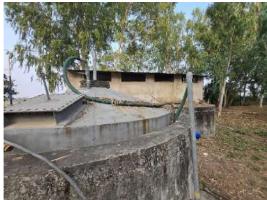
Fig.2: Biogas Plant Setup
